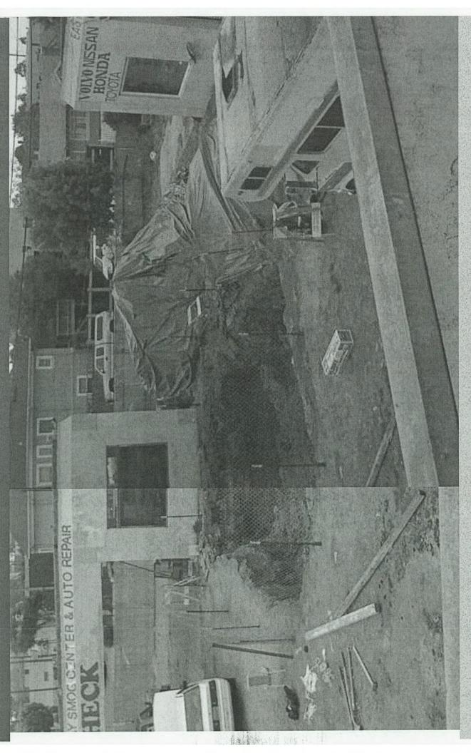
REMOVAL OF UNDERGROUND STORAGE TANKS WITHOUT PROPER PERMITS OR ENVIRONMENTAL OVERSIGHT work began late at night and without regulatory and environmental oversight as required by State law, which resulted in Site work stopped while Owner obtained permits / hired SOMA Environmental Engineers in 2010 strong toxic fumes in the area for weeks, endangering public health.
