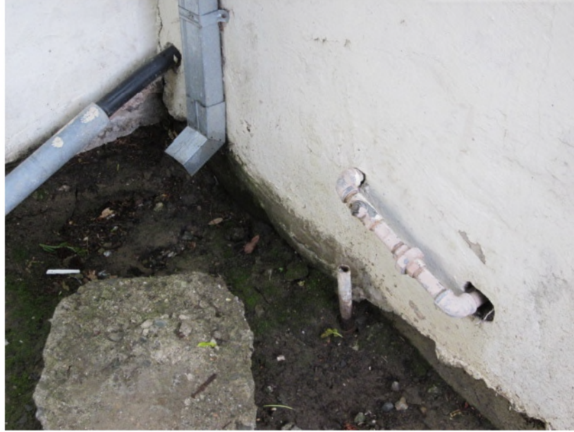
Photo 1. Exposed pipe on southwest side of Building 4. Cut-off pipe appears to be unused water pipe (refer to text).
