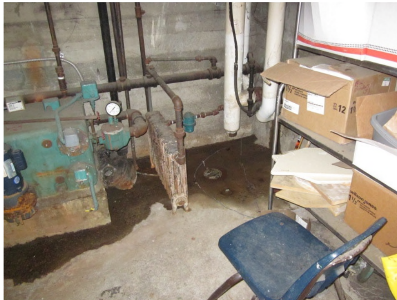
Photo 2. Water leakage in basement of Building 1.
