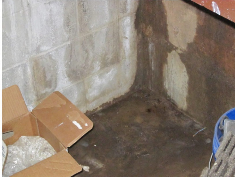
Photo 1. Water seepage in Building 5.
