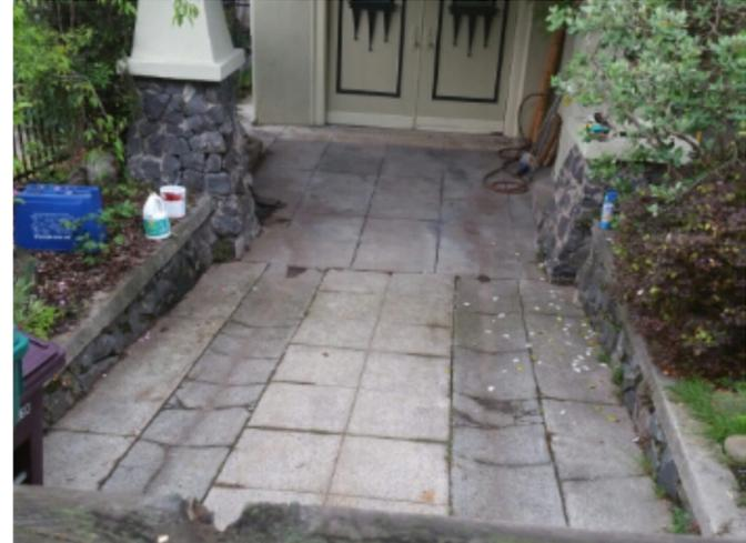
Cracks in concrete driveway seems like causing water intrusion to the basements. Concrete driveway requires repair or resurfacing.
