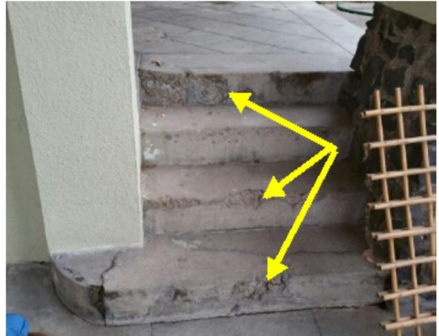
Concrete spalling on the front porch requires re-surfacing
