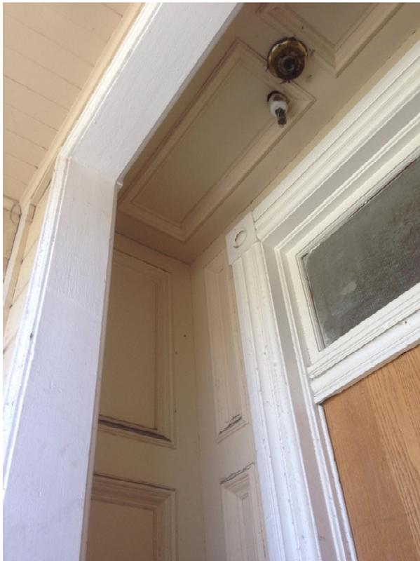
Original entry way, non-functional electrical and missing fixture.
