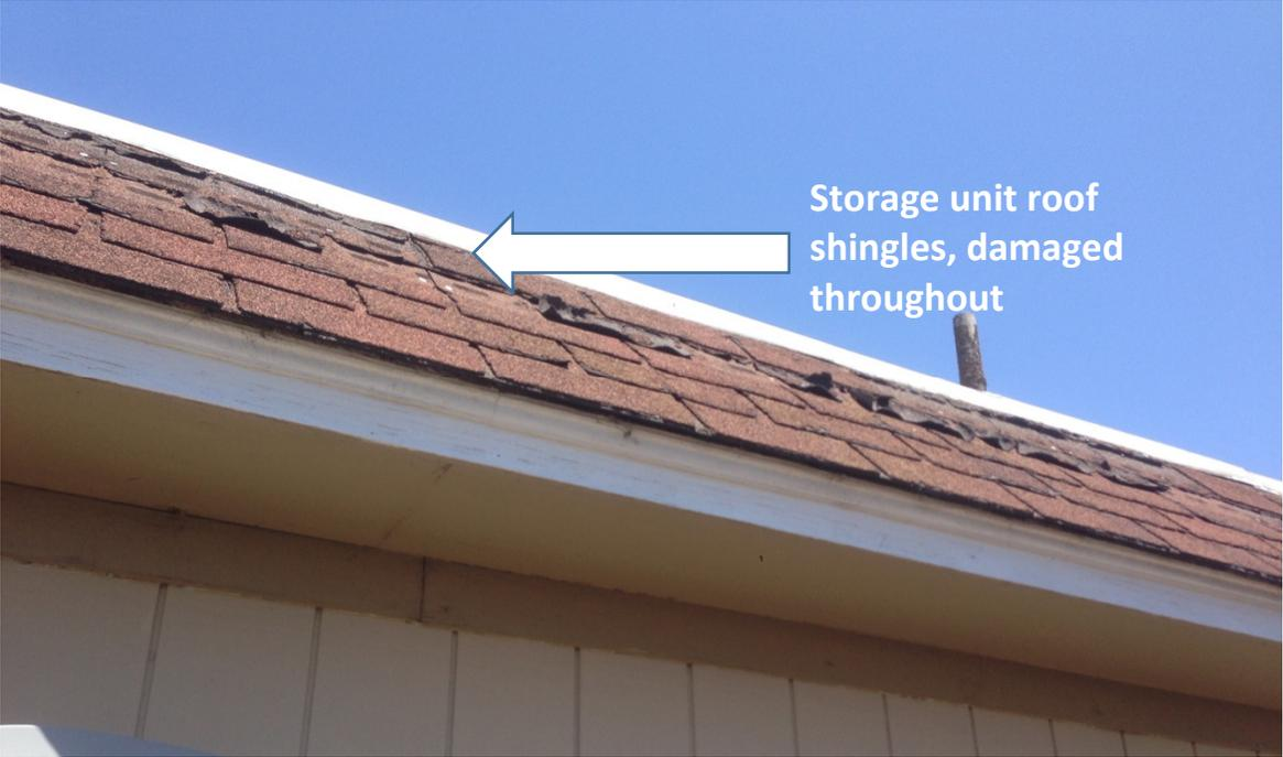
Storage unit roof shingles, damaged throughout
