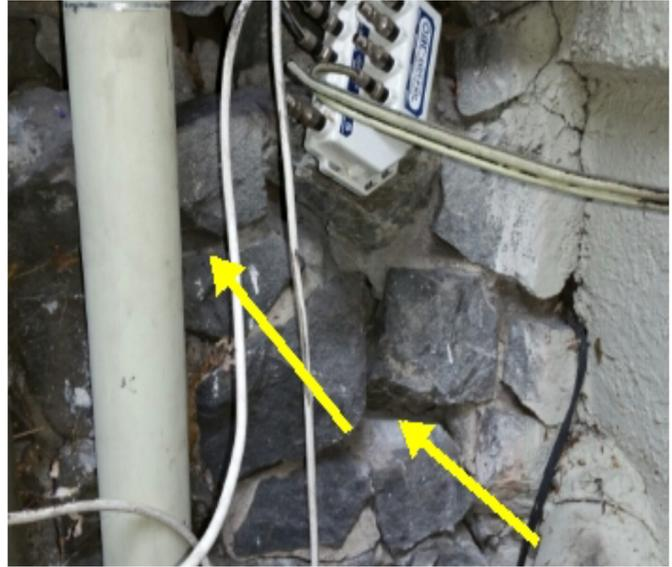
Water Intrusion in the basement in May 2017. Water intrusion in rainy months are severe and requires repair
