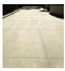
PEDESTRIAN PAVING - INTEGRAL COLOR CONCRETE WITH ROCK SALT FINISH, SAWOUT JOINTS
