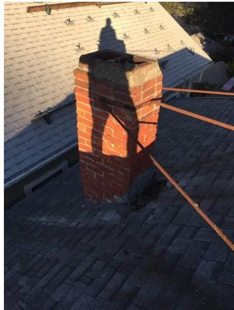
Repair brick chimney (currently a seismic hazard).
