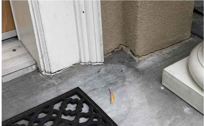
Work Program Item #1, Figures A and B: Separation of the concrete stairs from the residence foundation as a result of soil shifting to the rear slope (left). Sinking of the entry walkway and separation of the front porch as a result of general movement of earth to the west and south (right).
