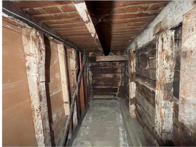
Work includes anchoring mudsills to the foundation, installing shear walls and shear transfer ties, and blocking in floor framing. Observe the absence of shear walls.
