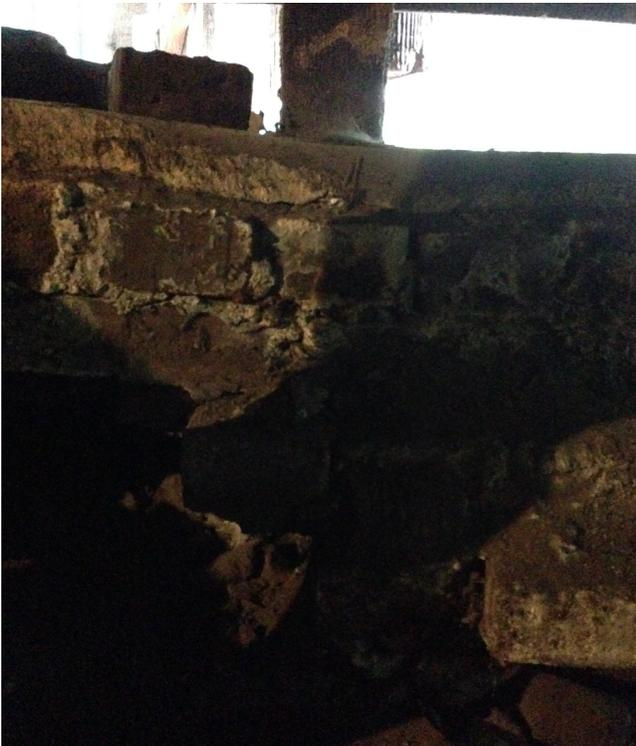
**Collapsing sill plate and hollowed out brick foundation**
