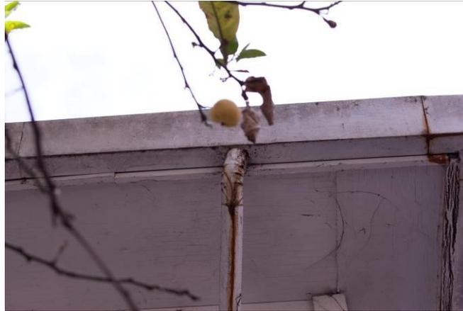
Replace roof and gutters. Repair, restore, and repaint rotten eaves, fascias, and ornamental woodwork at the eaves.
