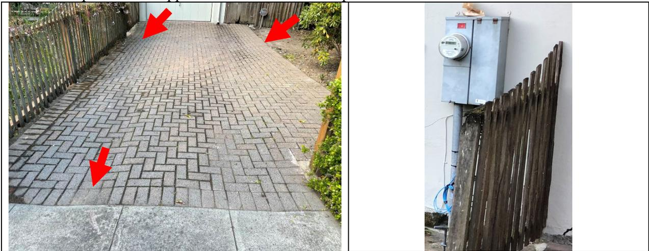
*Work Item #9 - Photo 1& 2 1990's era concrete brick driveway to be repaired. High spots and valleys are present. Sewer line underneath to be replaced. (If this was concrete it would be severely cracked but the brick helps conceal the soft sediment deformation. Exposed utility box.*
