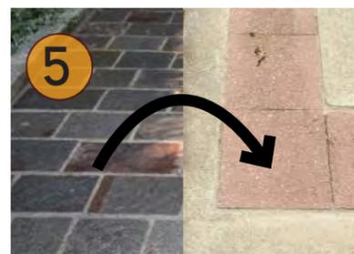
Stone Border; replaced by precast concrete paver
