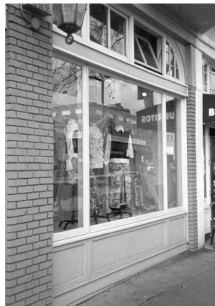
*2.1.8c Use standard projecting wood sills at wood and stucco bulkheads*
