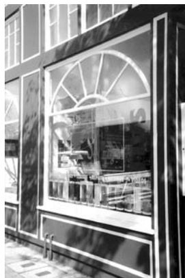
2.1.3b Use bulkhead materials and details which are compatible with facade walls and pilasters. Wood bulkheads are used in this example to complement the wood storefront.
