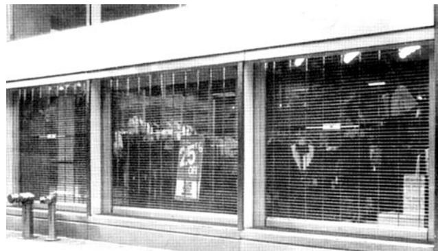
2.1.9a Use retractable grilles mounted behind the display window that are not visible during business hours
