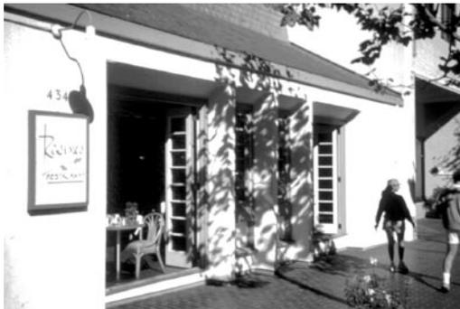
2.2.4c Folding doors used to open up full height of storefront
