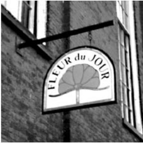
1.3.3a Simple round or square metal support brackets mounted to flush wall areas are appropriate in most cases
